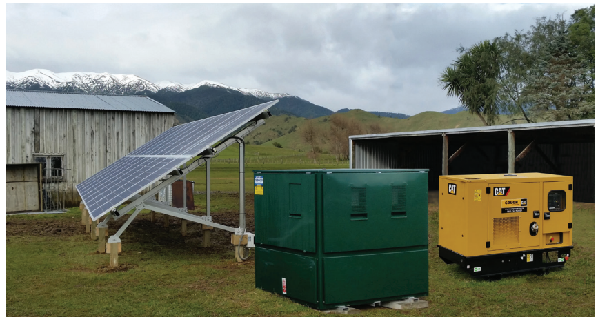
Base Power including the PV array, the Base Power unit, and the backup generator and fuel tank (From left to right)
