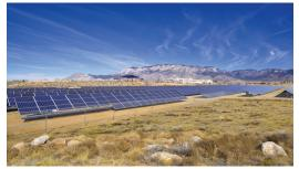
The Conext SmartGen Power System is a medium voltage power conversion substation delivering up to 4.8 MVA of solar power. It features two Conext SmartGeninverters, medium voltage transformer(s) and protection equipment. Cloud-connection and data collection enable remote diagnostics and servicing, as well as predictive maintenance.
